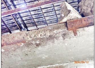
Multiple rigid frame columns have been dented and deformed
