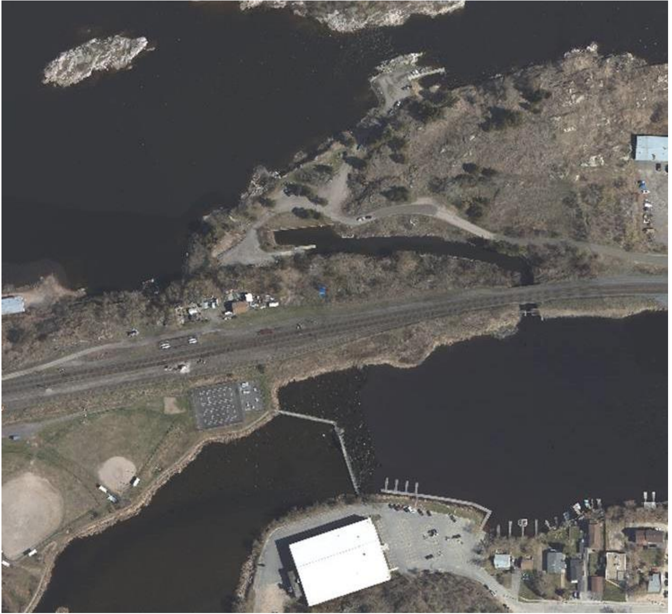
Figure 2 2023 Aerial Photograph of Keewatin Boat Launch/Portage Bay
